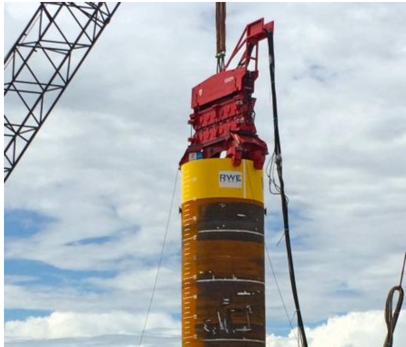
Figure 2-4 Clamping of vibratory hammer on top of a monopile 4
